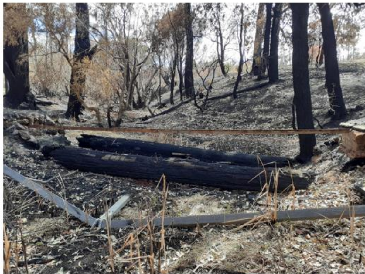
Tilden Park Footbridge
